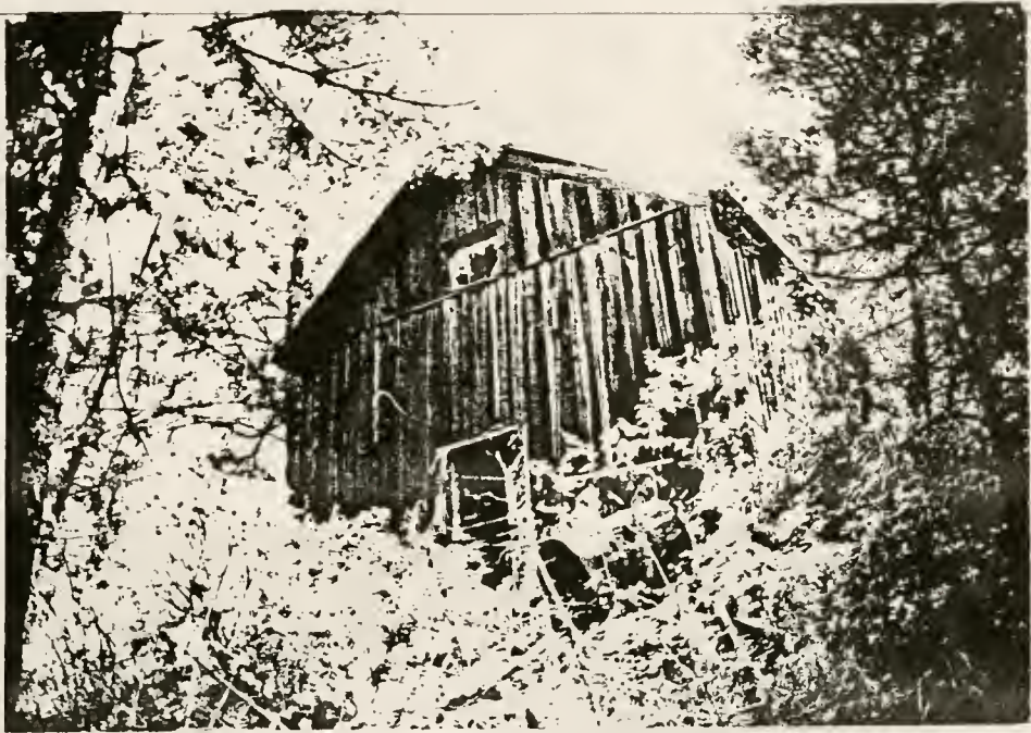
Figure 116. Structure #36, west side of water tank building.
